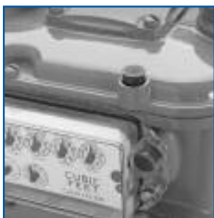
Screw is recessed in retainer collar then covered by replacement of security seal.
